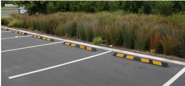
Resurfaced Parking lot with enhancements
