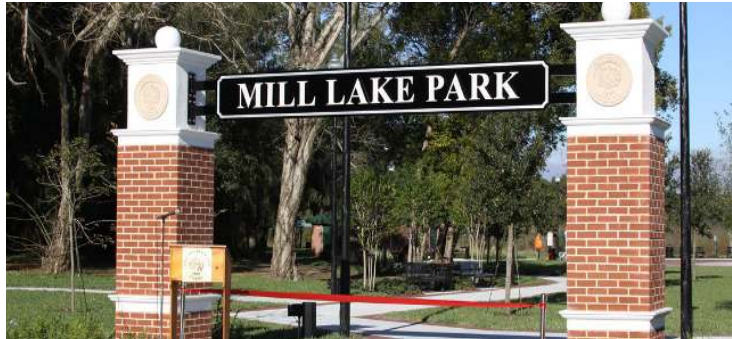
Overhead Gateway Signage
