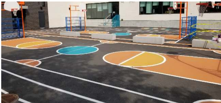
Coloured Concrete Surfacing
