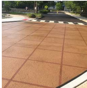
Change in Surfacing/ Paving
